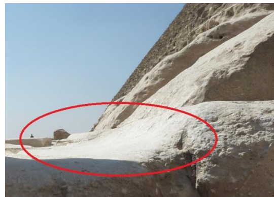
Fig. 3 Uniform erosion on limestone rock.
