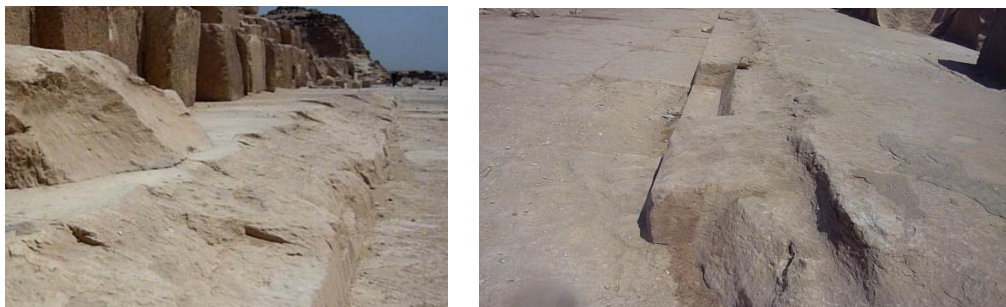
Fig. 16 Wear or erosion of the paving immediately outside the cladding blocks at point 8, and, in Fig. 17, at point 9.
