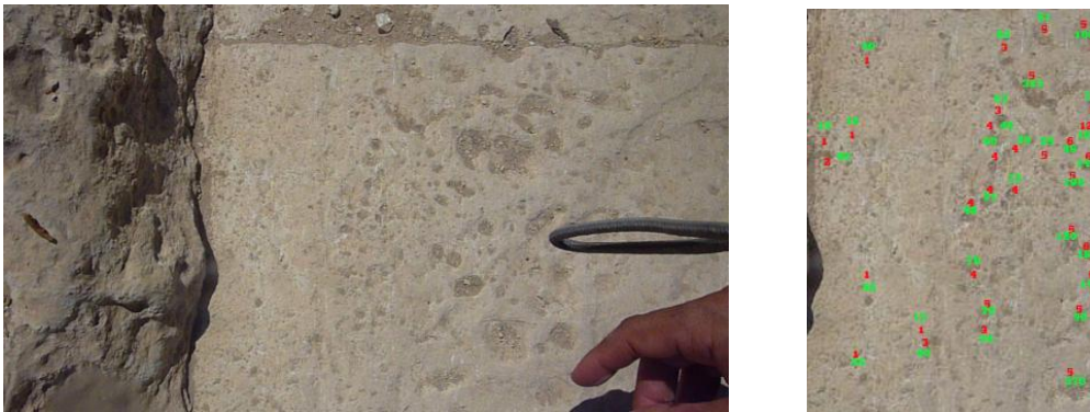
Fig. 20 The difference in erosion at point 12 between the right side (which has been exposed since the pyramid was built) and the left side.
